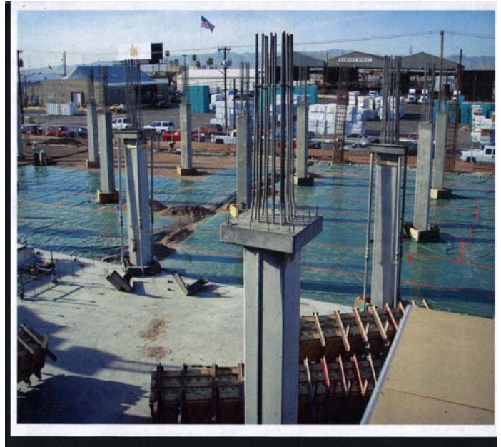
July 07. Preparing the first floor for an all-night concrete pour.
