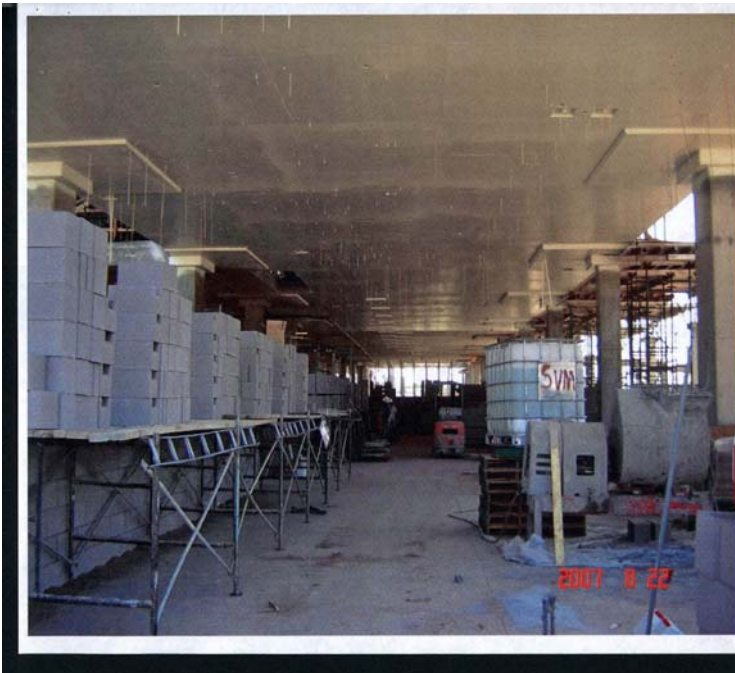
August 22, 07. Concrete Block stacked on the first floor.
