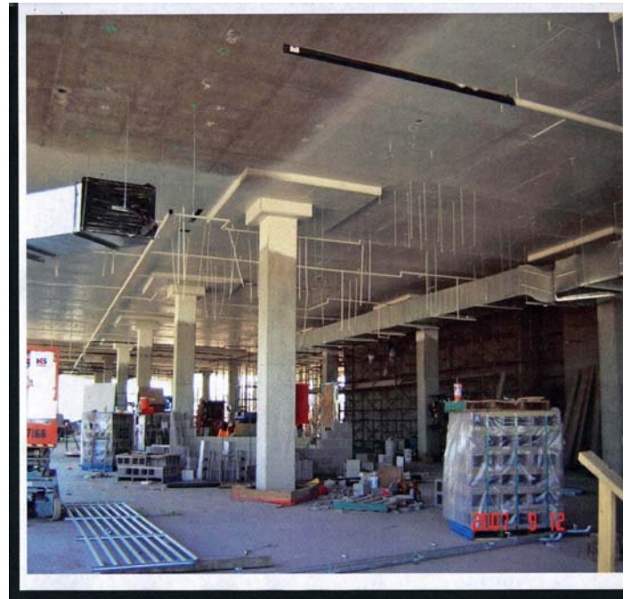
September 12. 07. Hanging ductwork from the ceiling.
