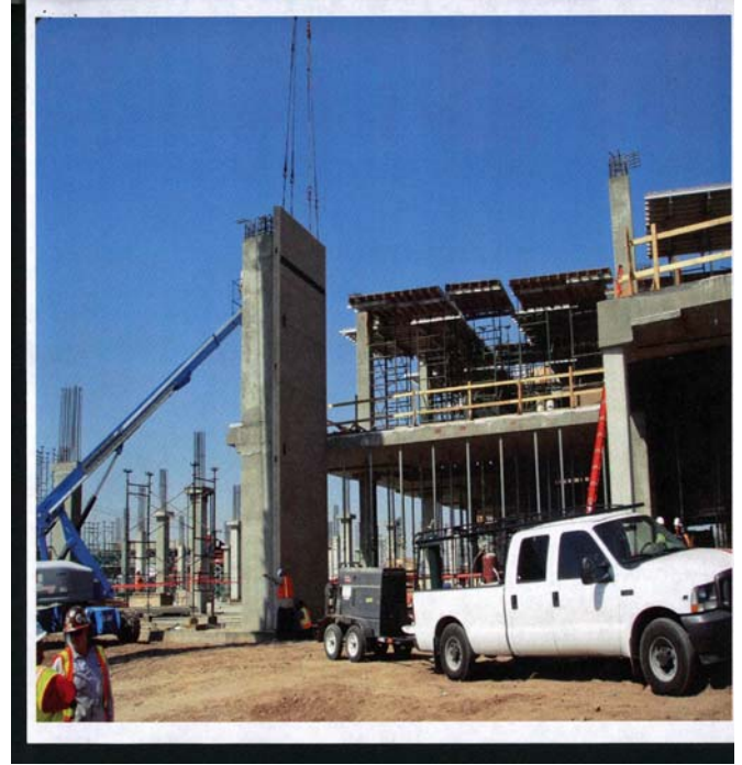
August 07. Attaching a pre-fab piece onto a foundation column.
