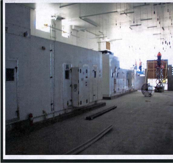
September 07. Flash-freeze isolation rooms. The fan is curing concrete.
