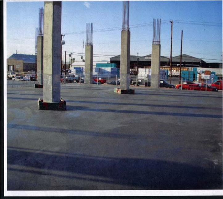
August 07. Fresh concrete after pouring all night.
