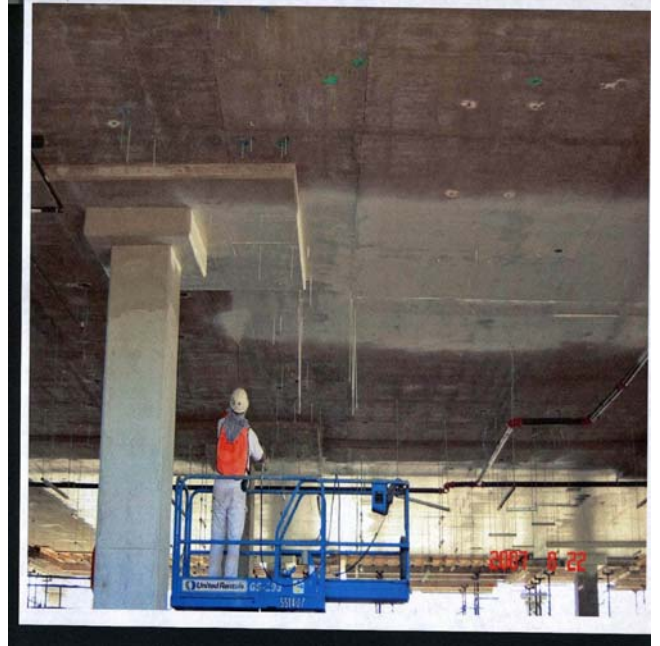
September 07 Spraying sealant underneath the top floor
